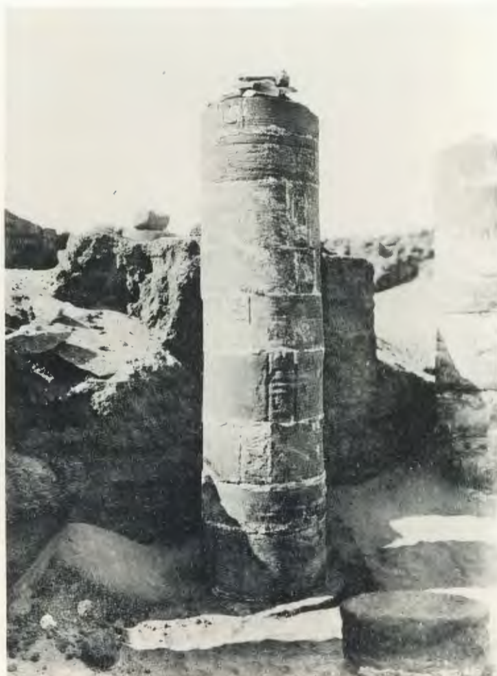
d. Column 4 from SE.
