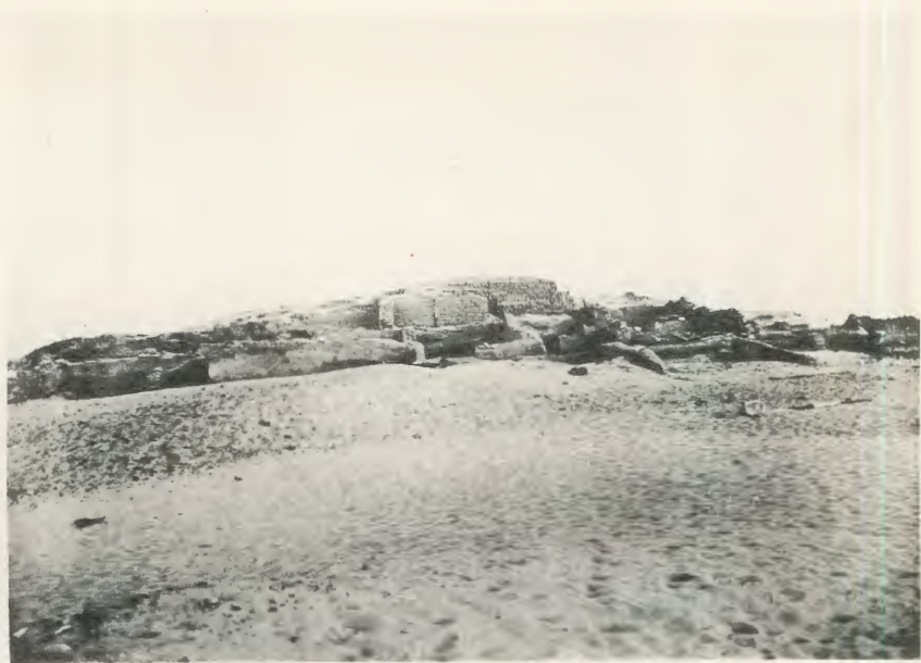
b. From W., after excavation
