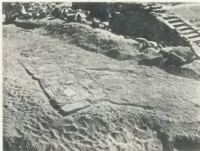
d. Flag and rubble paving to N. and NW. of Altar (1935-6)
