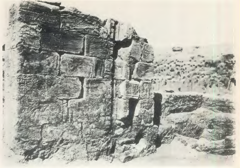
b. Entrance to 1st Court, W. side of door, showing swing-marks
