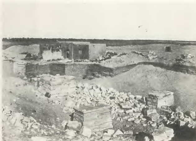
d. Site III. Meroitic curtain wall from SE.
