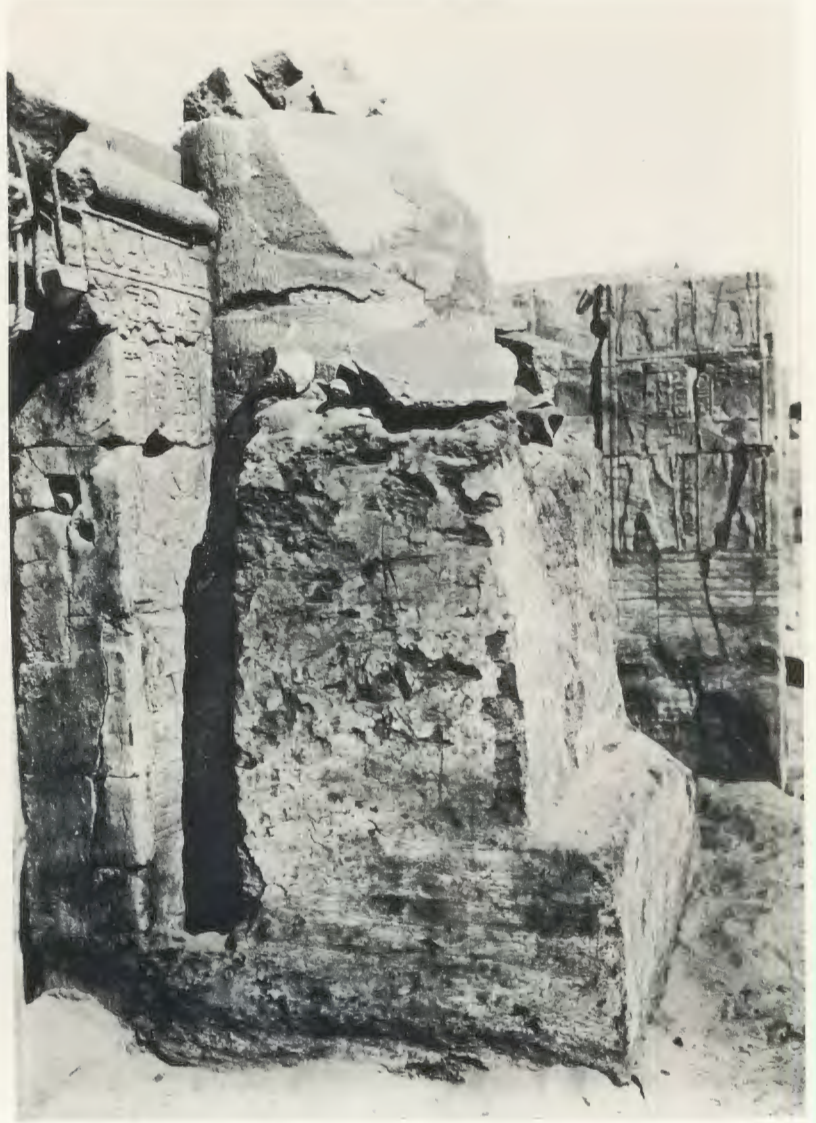
b. Brick structure, W. side (1930-1)
